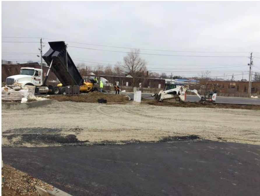
Project Site on March 20, 2019 View of the parking lot and installation of the asphalt binder course.
