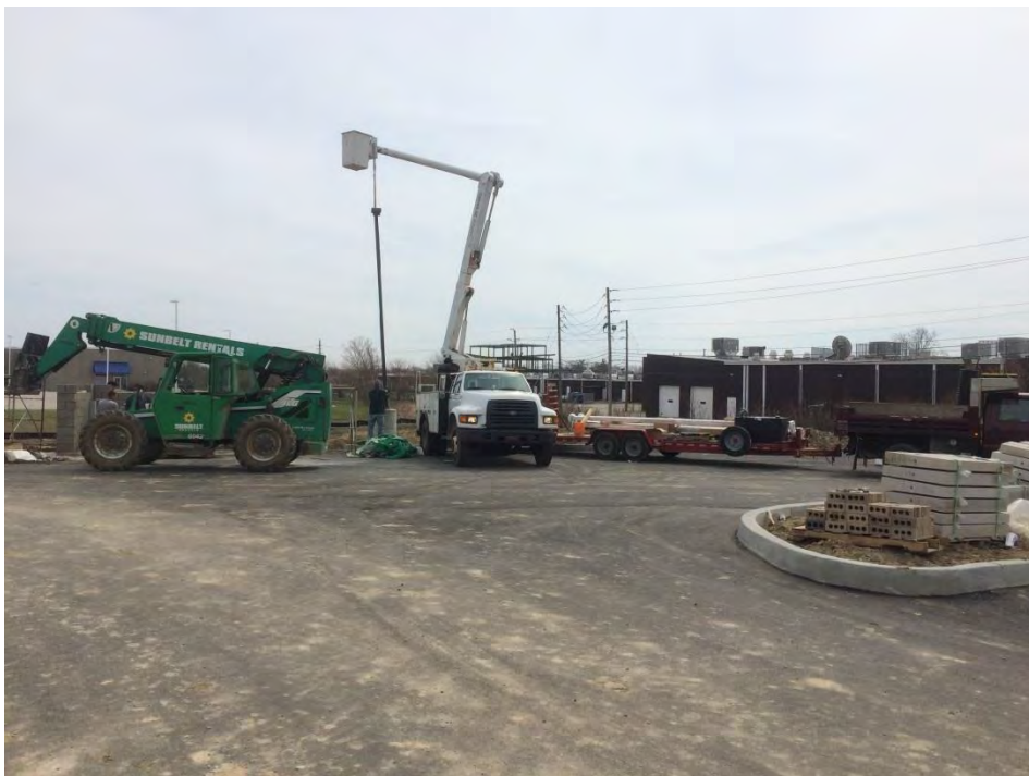
Project Site on April 4, 2019 View of the installation of the site lighting.
