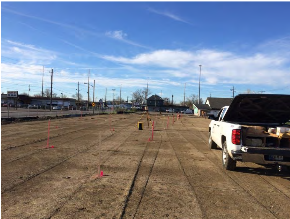
Project Site on March 26, 2019 View of the building pad with staking and layout in process.
