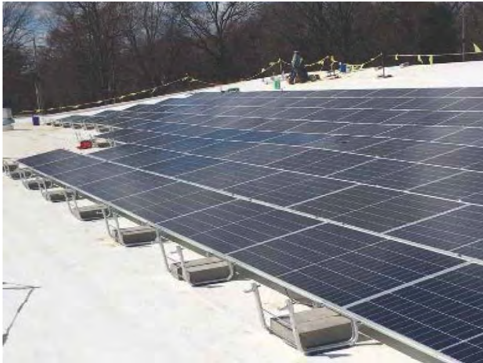
Project Site on March 26, 2019 View of the installed solar panels on the roof.
